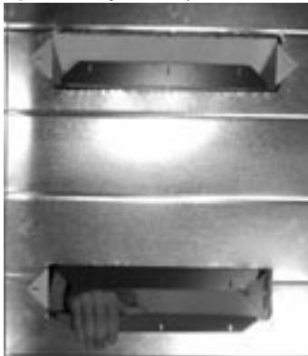
figure 2.3b - Unfold the ducting flaps completely to sandwich the return air plenum between the ducting flaps and the filtration unit.
