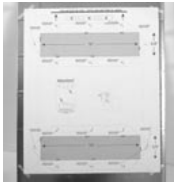
figure 2.1a - Tape template to return air plenum. Cut opening with metal shears and predrill for the securing screws.
