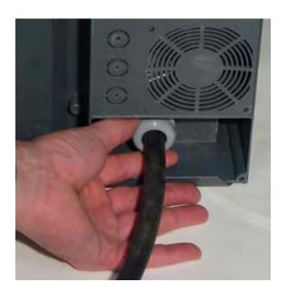
Connect power wires into terminals N and L. A green/yellow ground terminal (which is also the chassis ground) is provided for connection of the ground wire.
