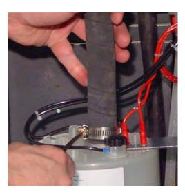
WARNING: the length of the steam hose should be less than 12 feet.
